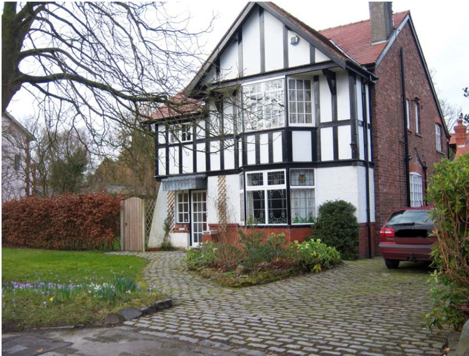
One of the original Edwardian properties displaying a number of original features.
